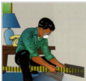
The most effective way to clean air ducts and ventilation systems is to employ Source Removal methods of cleaning. This requires a contractor to place the system under negative pressure, through the use of a specialized, powerful vacuum. While the vacuum draws air through the system, devices are inserted into the ducts to dislodge any debris that might be stuck to interior surfaces. The debris can then travel down the ducts to the vacuum, which removes it from the system and the home.
